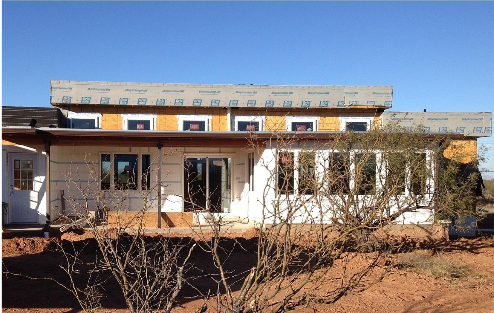
High reflectance & emissivity roof coating
